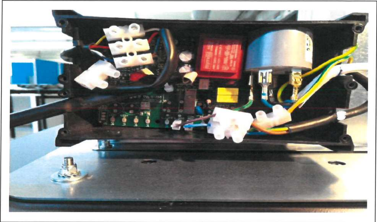
No.5 Internal View
